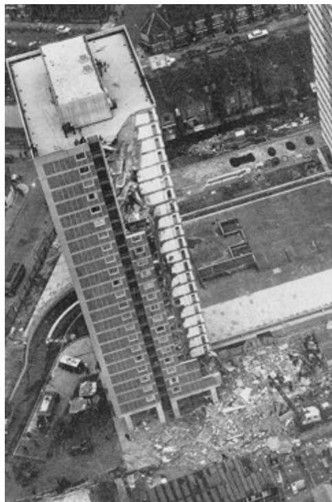
Figure 1.1: Ronan Point Building following partial progressive collapse in 1968. (Photo: UK Crown Copyright)
