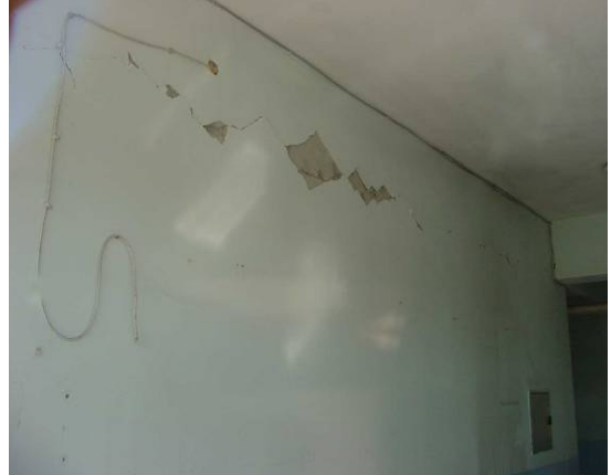
Figure 4. Rekabet Kurumu High School after 2003 Bingol Earthquake (Light)
