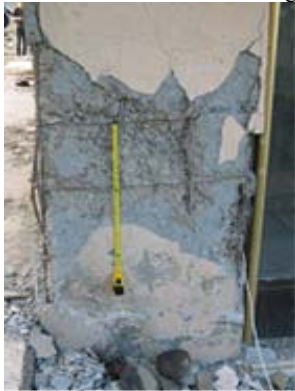
Column detailing in plastic hinge region
