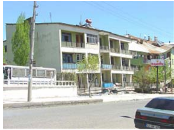
Ground story collapse of 4-story building
