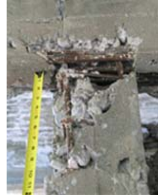
Beam column joint in building under construction
