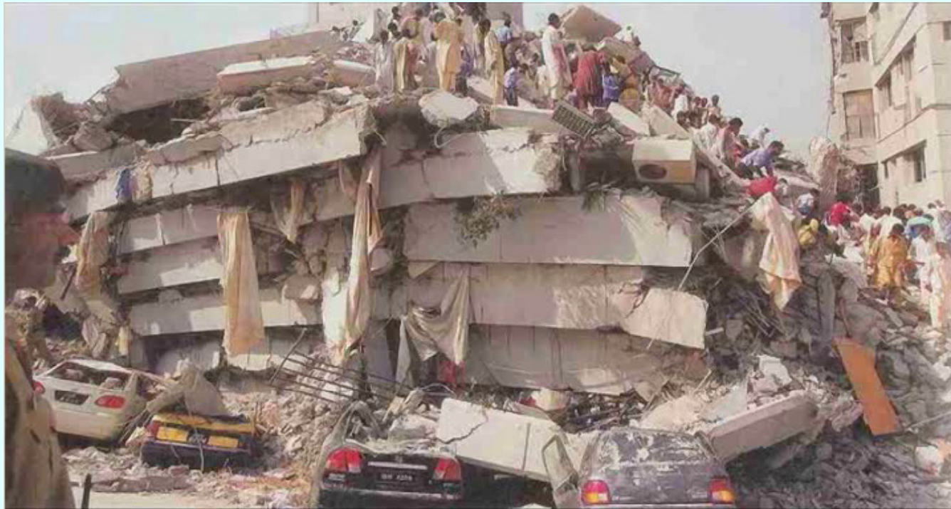
pancake-type collapse of a 10-story building triggered by an earthquake (Islamabad, 2005)
