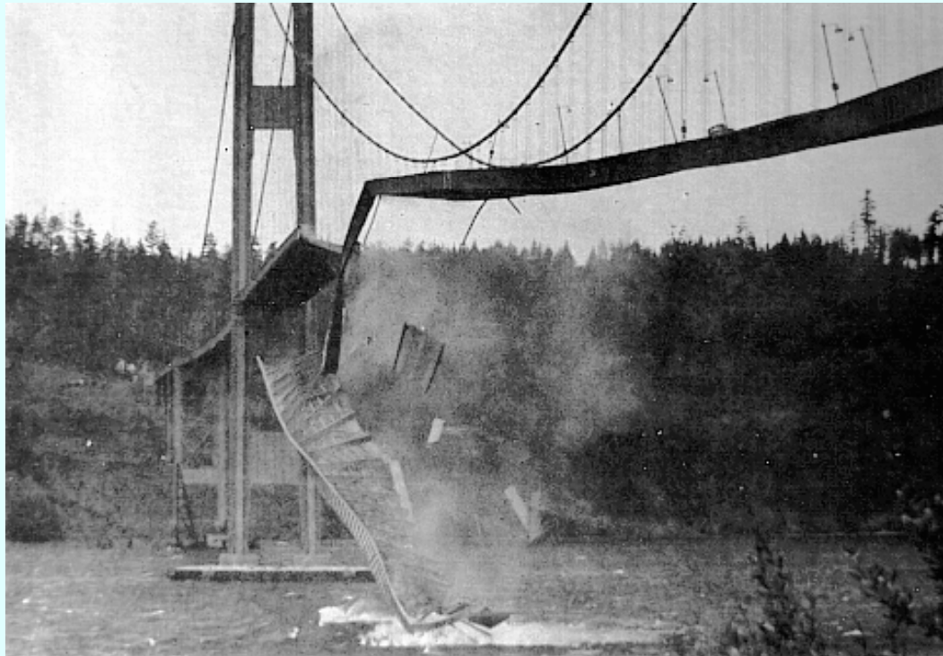
zipper-type collapse of the Tacoma Narrows Bridge triggered by wind-induced vibrations (1940)
