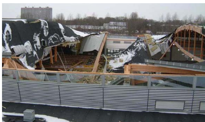
a) An intact truss is seen to the right
