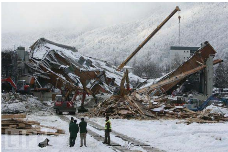
Figure 3: Bad Reichenhall ice-arena collapse
