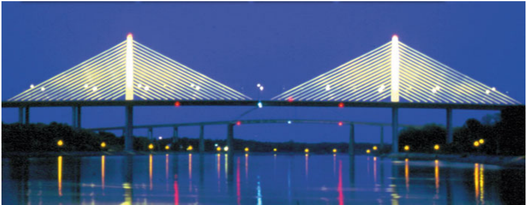
Chesapeake-Delaware-Canal Bridge, USA
