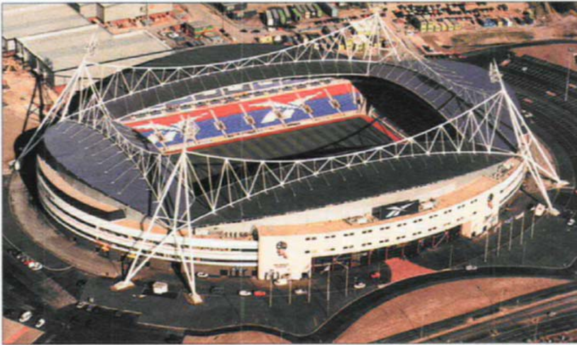
Fig. 1: Aerial view of the stadium
